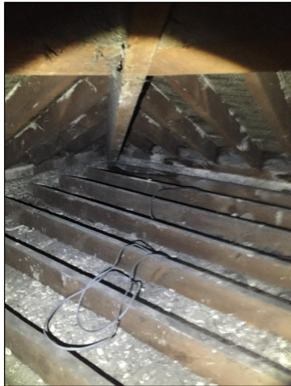
Plate 6: Internal attic space in Craigmole House. White debris is lime rendering.
